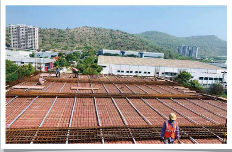
RYAN SCHOOL- 7th slab work is in progress
