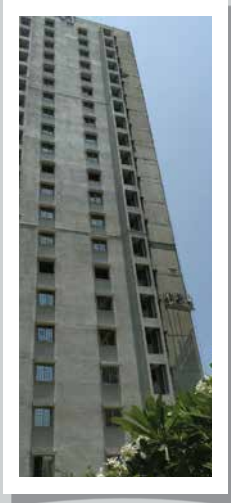
PALLADIO-E - West side surface preparation work is in progress
