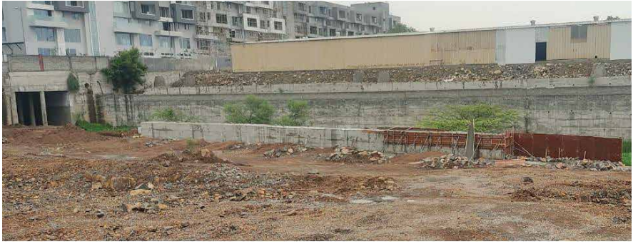
YO- North east corner compound wall work is in progress
