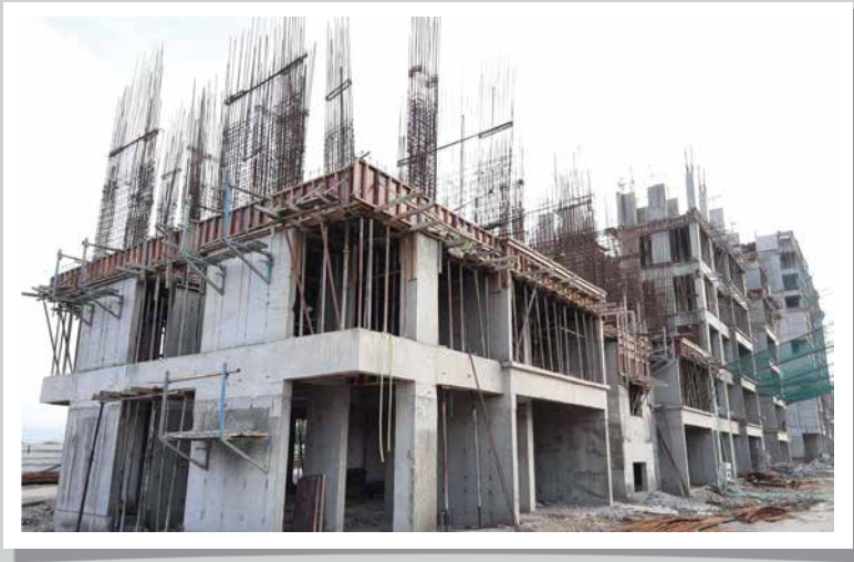
YSNW-D- 3rd floor shearwall reinforcement has been completed
