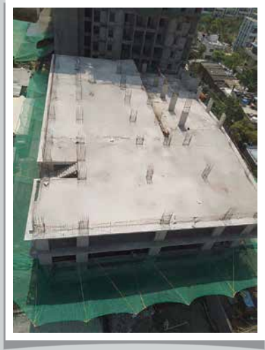
Y1WC-E- 5th slab casting work has been completed
