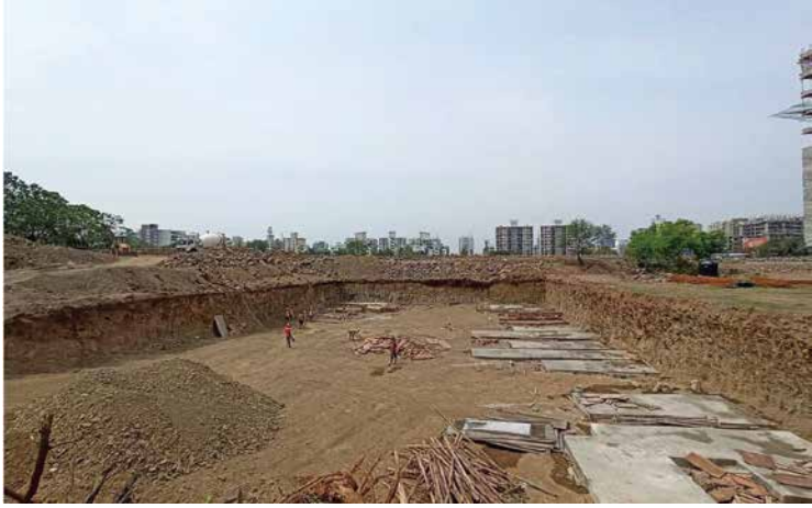
YSN-A- PCC work is in progress
