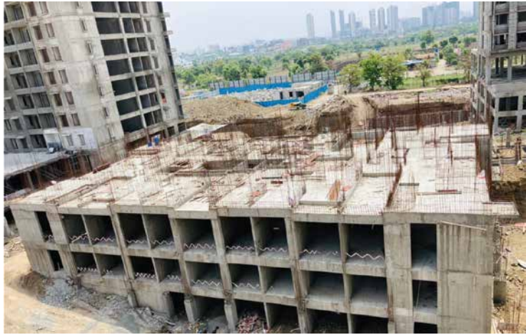
Y1H-D- Lower parking, upper parking & 1st floor slab has been completed
