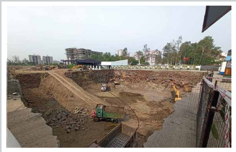
VJTC- Excavation work is in progress
