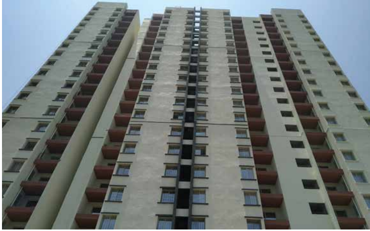
PALLADIO-E - South side 2nd coat external paint work is in progress
