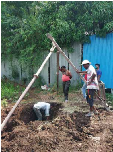
YO- South side compound wall column pile work is in progress
