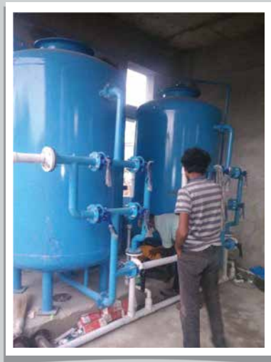
YE-STP- Plant installation work is in progress
