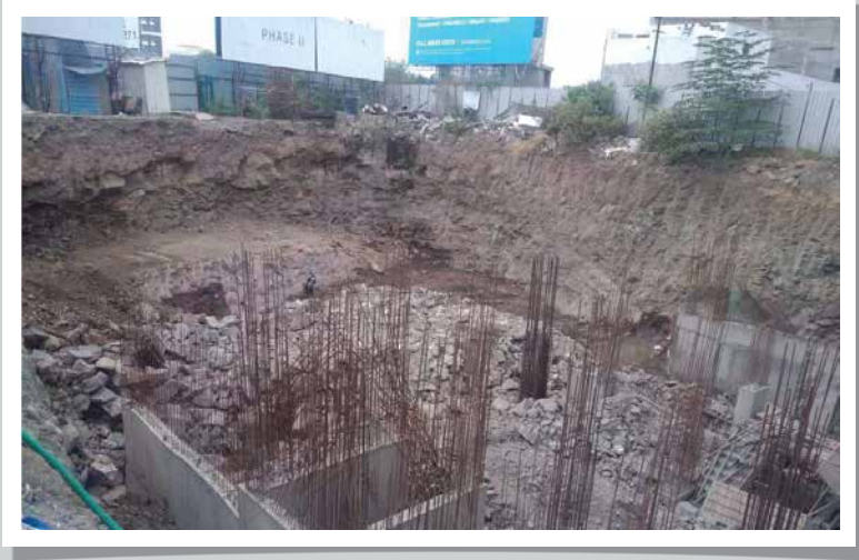
YE- Commercial building excavation work is in progress
