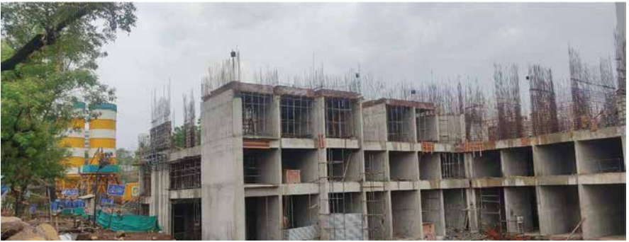
YO-B- 3rd slab shuttering work is in progress
