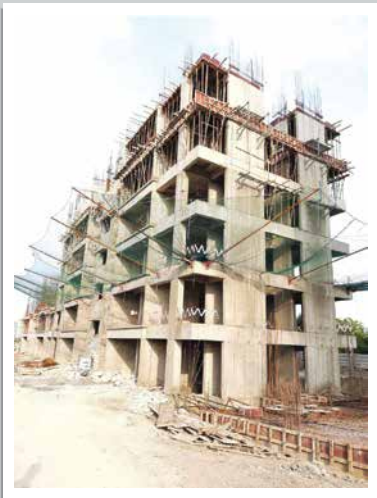
YSNW-C- 6th floor slab shuttering work is in progress
