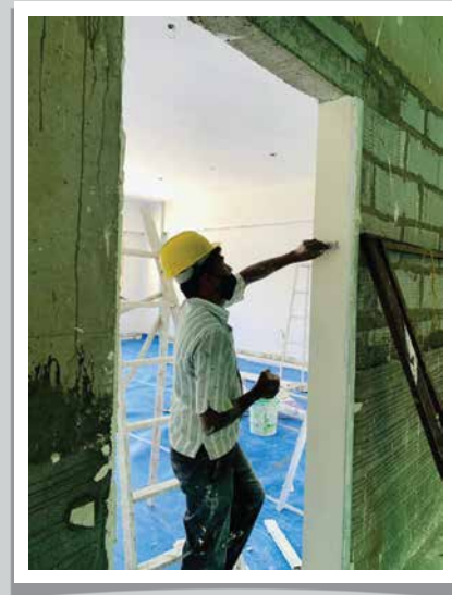
RYAN SCHOOL- Gypsum work is in progress on 3rd floor
