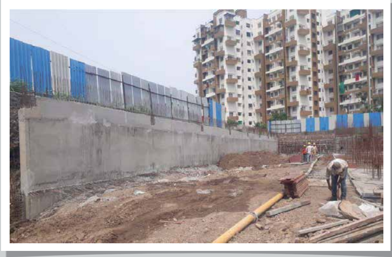
Y1In-D1D2- Retaining wall casting work is in progress
