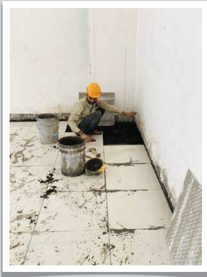
RYAN SCHOOL- Tile work is in progress on 2nd floor
