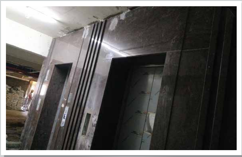
PALLADIO-E - Lift cladding work for passengers lifts has been completed
