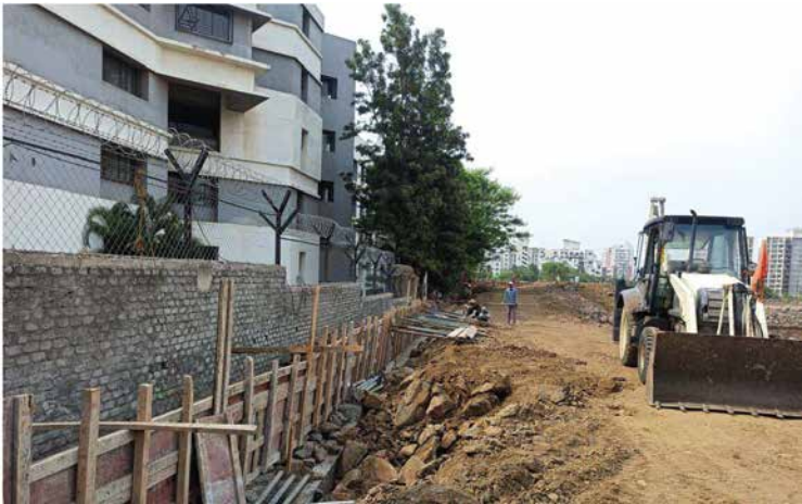
YSN- Retaining wall work is in progress
