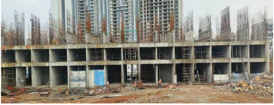
YO-A- 2nd slab shuttering work is in progress
