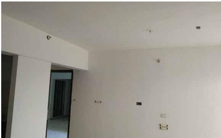
PALLADIO-E - 1st coat of internal paint work is in progress
